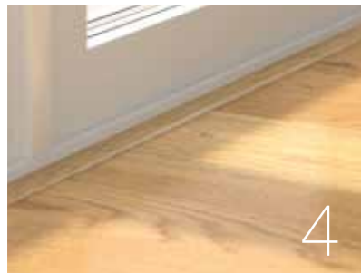
End moulding Finishing up to threshold, sliding doors, etc
