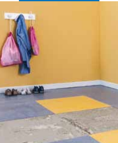
Removing a portion of resilient floor covering in the area to be repaired
