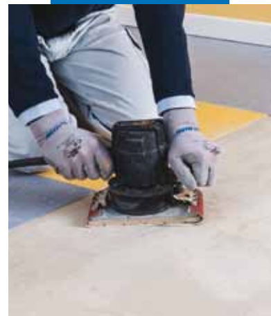
Grinding after 2 hours
