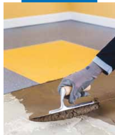
Skimming the substrate to a feather edge
