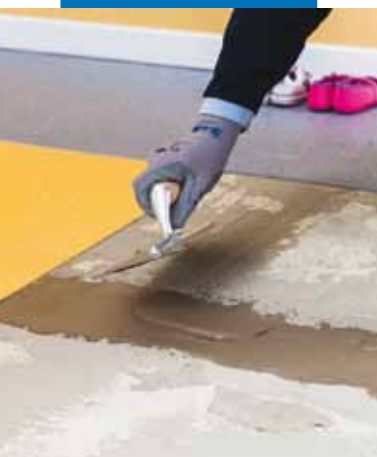
Reintegrating a portion of the substrate
